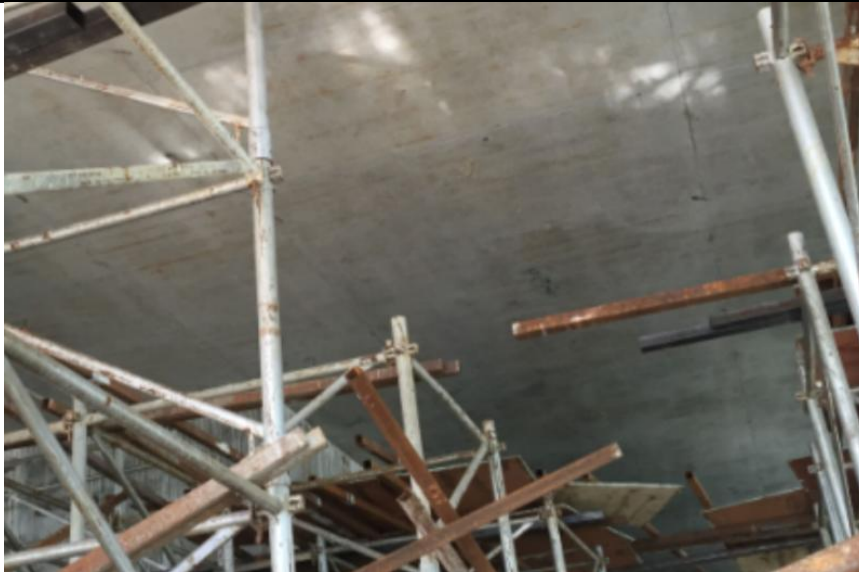
Figure 6: Demounting status of 1000mm board on A7 floor.
